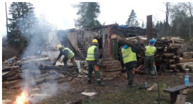
Men taking-down the building
